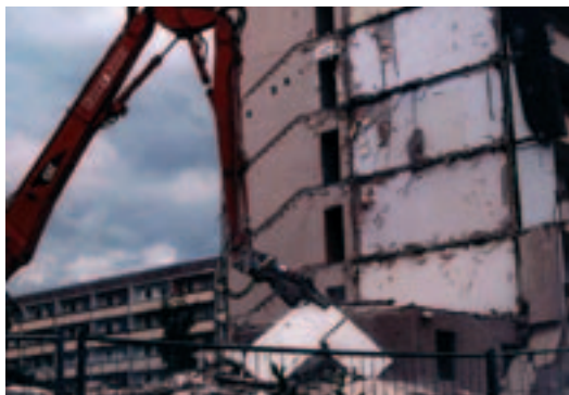
Cautious removal with a gripper-like demolition tool
