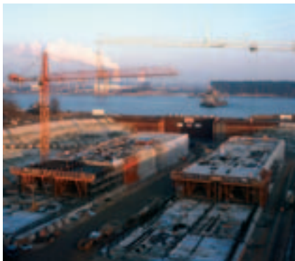
Prefabrication of two tunnel elements in the dock beside the river (courtesy of Heinrich Hirdes GmbH)
