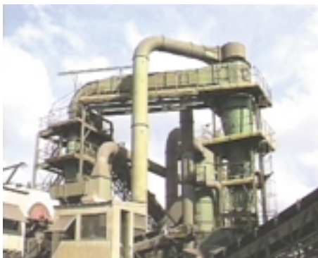
Example of a dust-sucking and cleaning device co-financed by a CRAM in a crushing centre for the cleaning up and recycling of metals.
