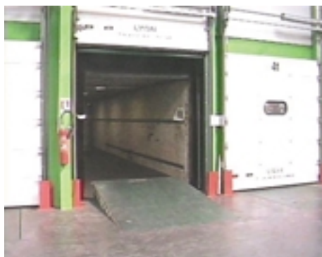
Example of a working station in a transportation company co-financed by a CRAM: platform able to adjust itself to the various type of trailers.
