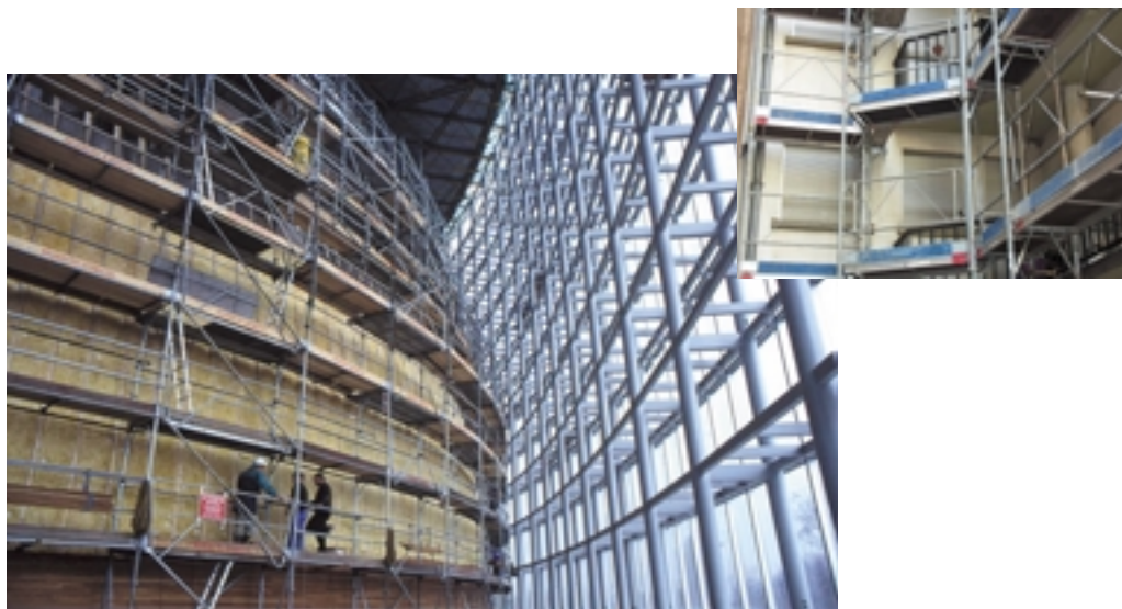
Below: Scaffolding in the European Parliament construction site in Strasbourg.
