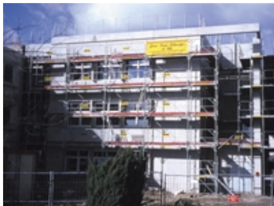
General view of an office building under construction.
