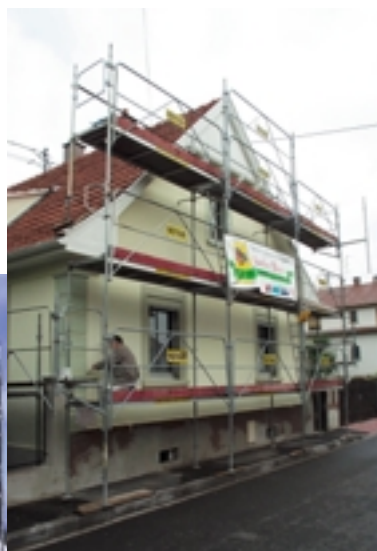
Above and next page: scaffolding that can be assembled safely for private dwellings.
