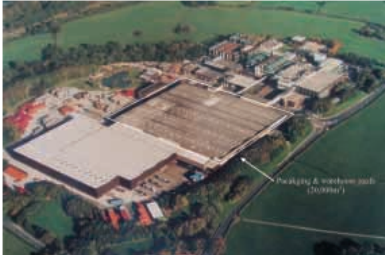
Aerial view of the work area
