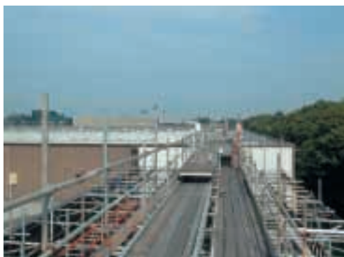
Materials loading scaffold & roof trolley system
