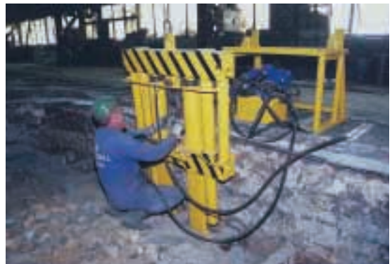
Work carried out using the hydraulic pulling machine
