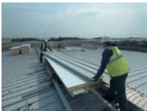
Laying of new roof sheets
