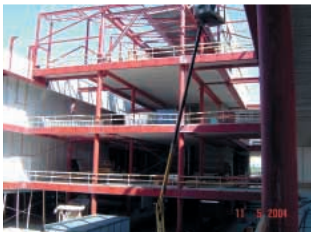
'The ever changing construction site'
