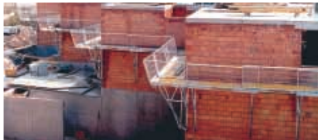
Scaffolding in use
