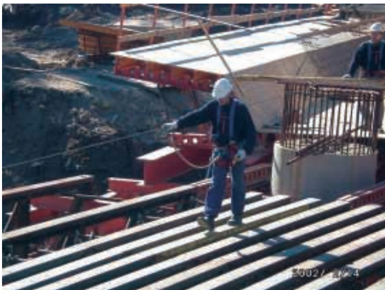
Use of fall arrest equipment, before edge protection is in place.
