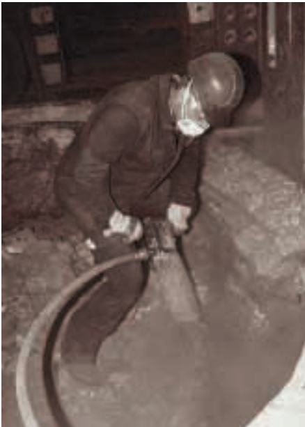
Old method using power hammer
