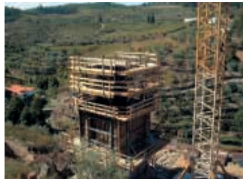
Bridge under construction
