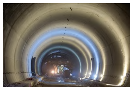
Tunnel T1 during construction
