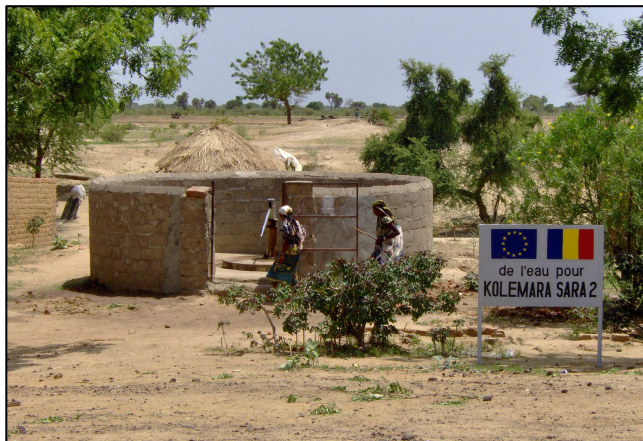
Waterhole construction in Kolemara Sara, Chad
